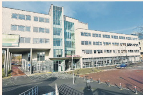
Stationside 2 van City Side Apartments in Apeldoorn. FOTO: CSA
